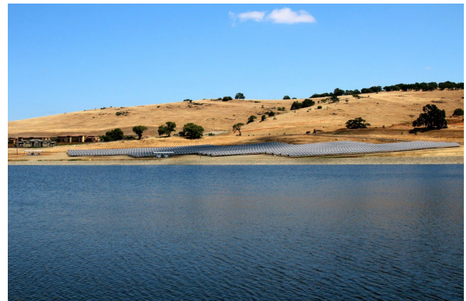
El Dorado Hills Wastewater Treatment Plant Storage Reservoir and Solar Plant
