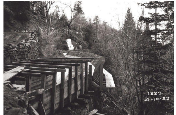
Flume under construction in 1923
