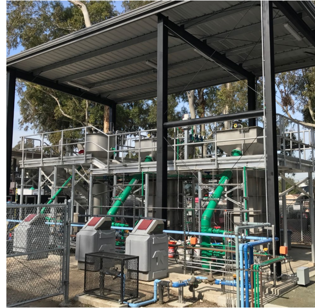
Demonstration -scale SAF-MBR (24,000 gal/d)
