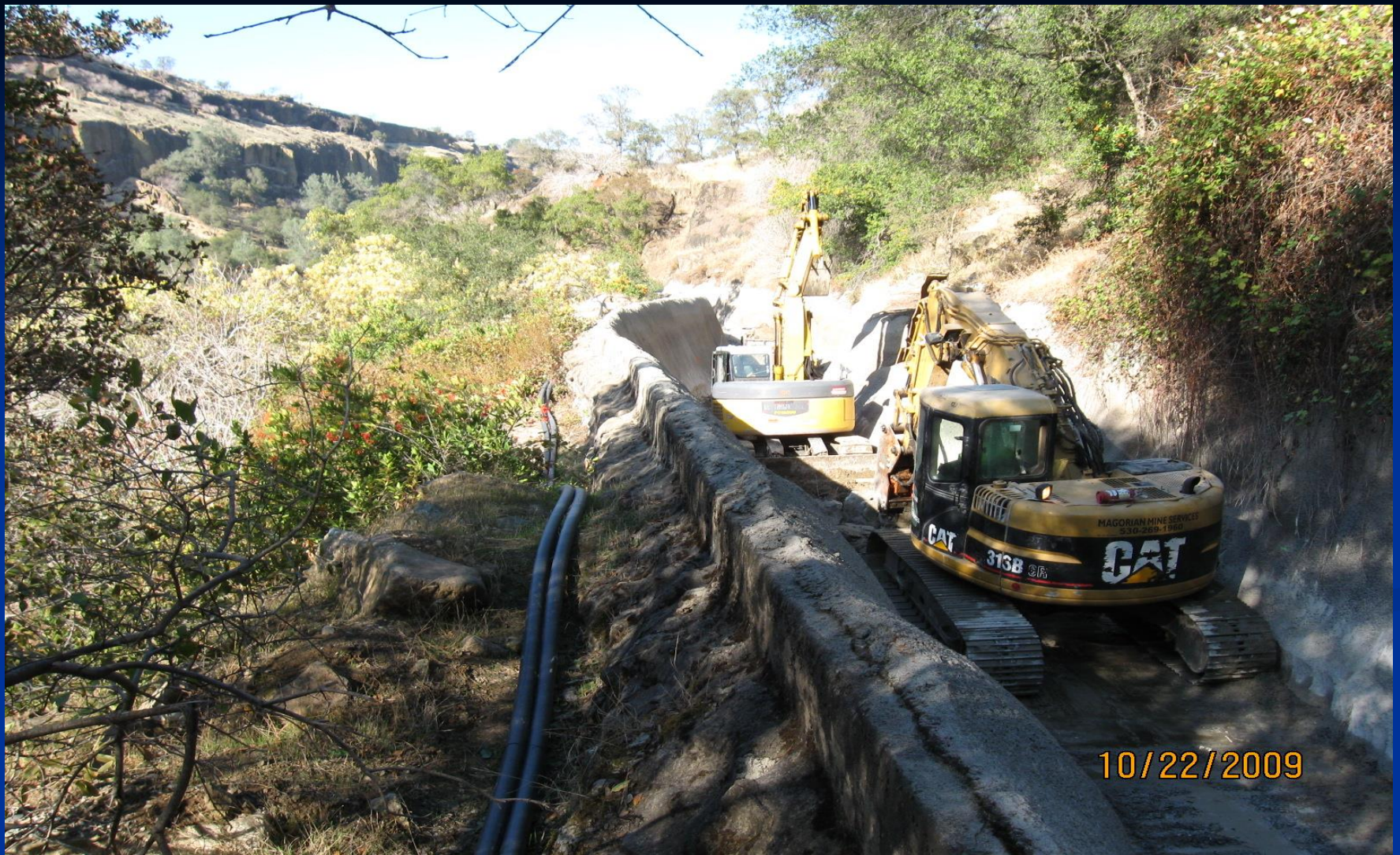
Segment 1: Canal Invert Demolition in Structural Rehab Area
