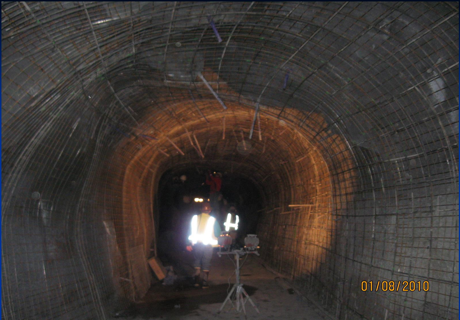
Segment 1: Tunnel 4 Repair in Thin Cover Section – Wire Mesh and Reinforcement Installation
