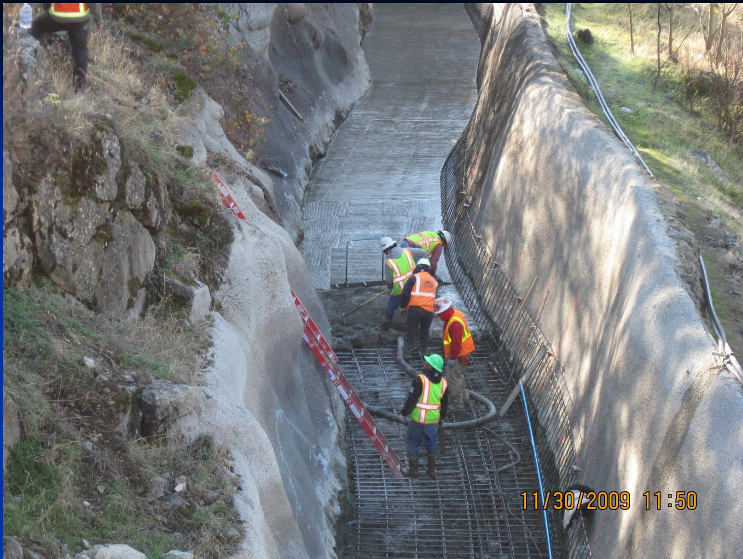
Segment 1: Structural Invert Concrete Placement After Micro-Pile Installation
