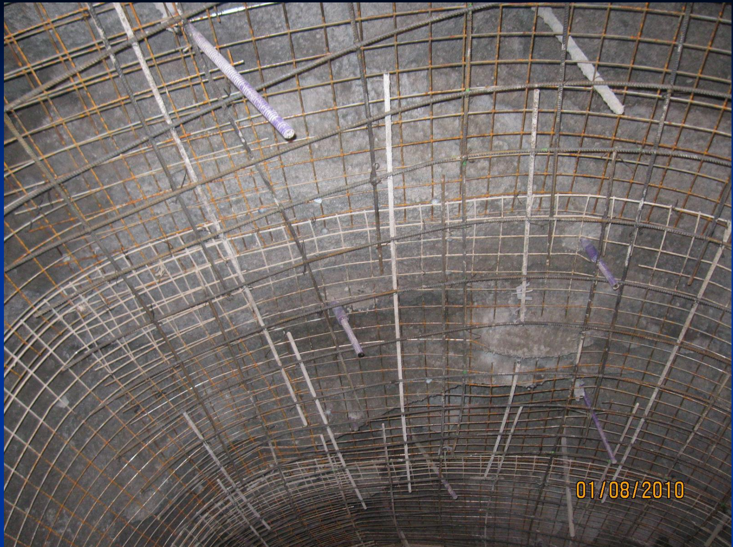
Segment 1: Tunnel 4 Repair in Thin Cover Section – Wire Mesh and Reinforcement Installation
