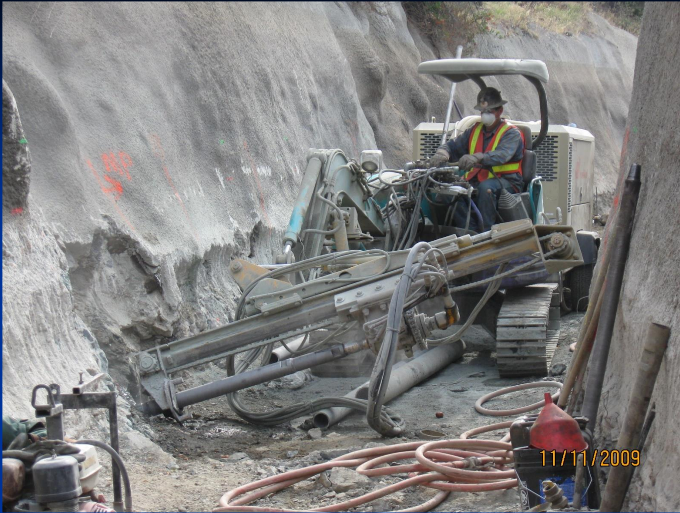
Segment 1: Canal Invert Lateral Tieback Installation in Structural Rehab Area
