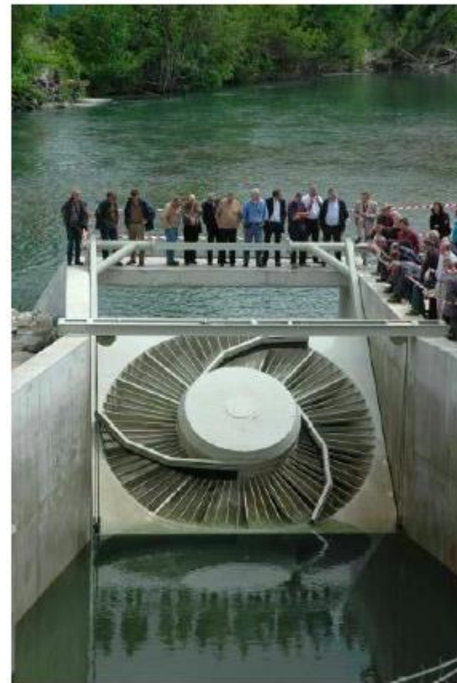
VLH in Withdrawn Maintenance Position
