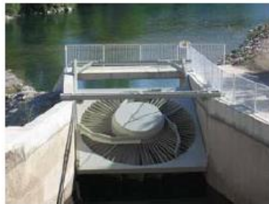
VLH in Withdrawn Maintenance Position
