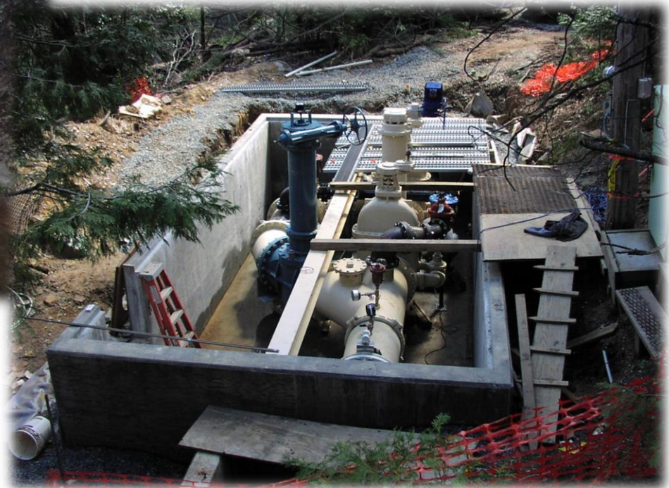
Terminus of Gold Run Pipeline (PSV)
