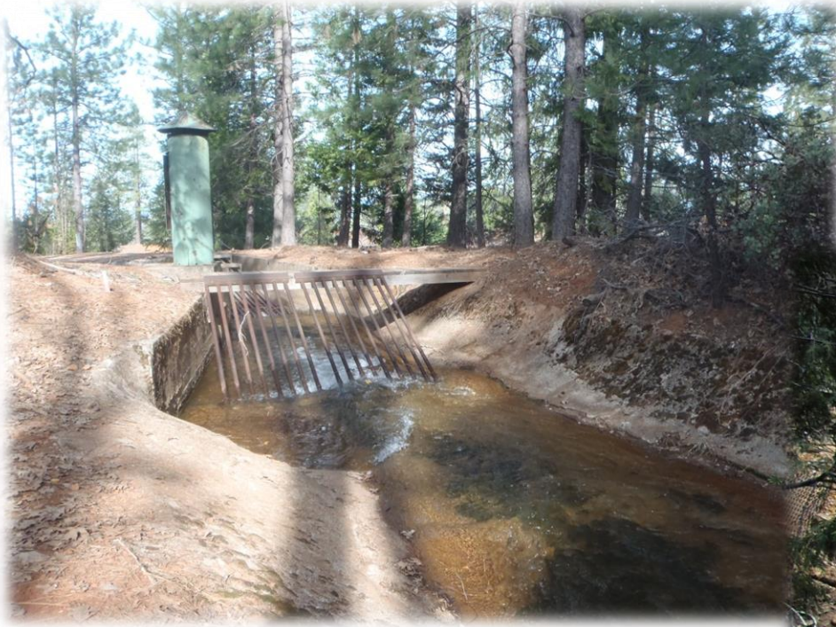
Inlet to Gold Run Pipeline
