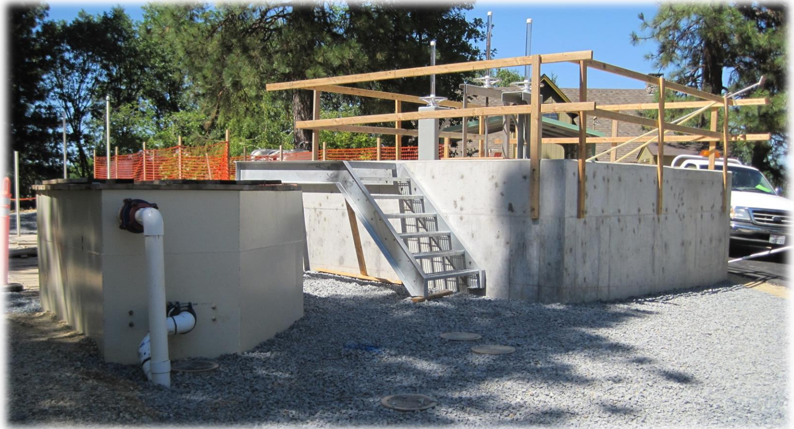
Outlet Structure (Colfax Header Box)
